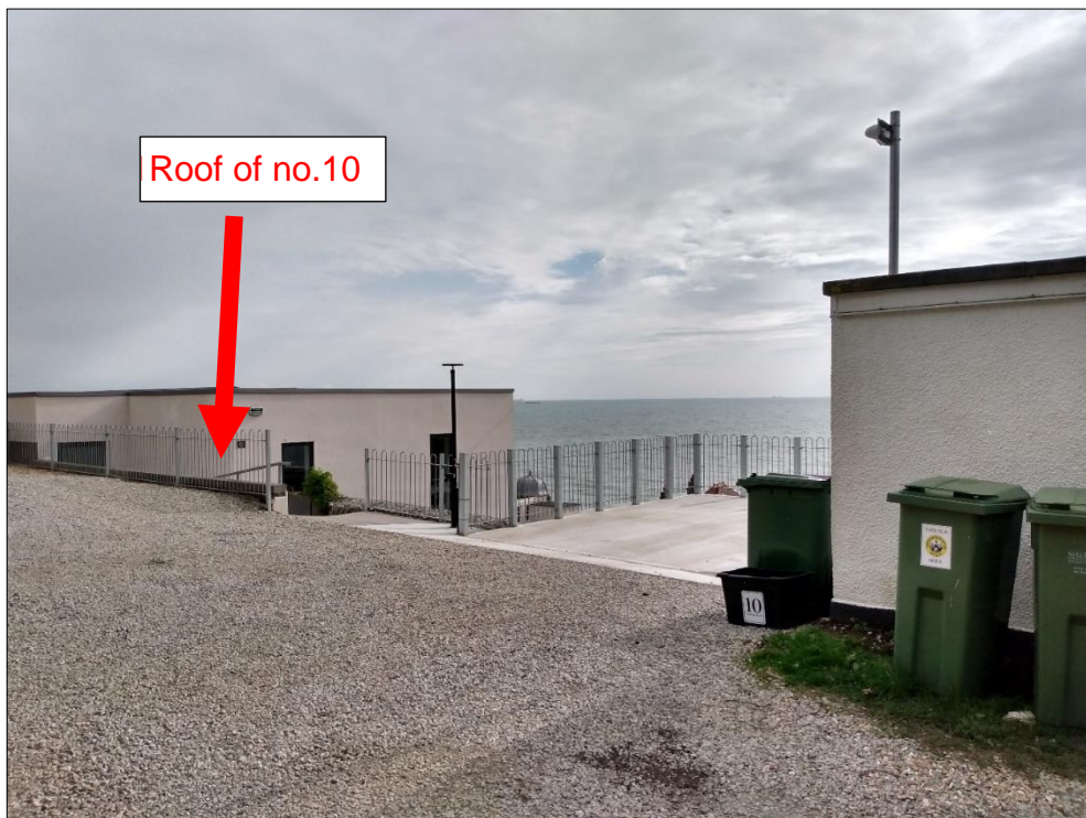
Figure 4: Parking area, neighbour's garage, and no.10.
